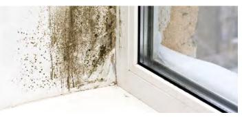
Well-made modern windows have a much better sealing and thermal insulation properties than their older counterparts but this however prevent the air and humidity from crossing through cracks and crevices. The result of airtight windows is a dramatically changed indoor climate because the concentration of harmful gases, humidity and CO<sub>2</sub> can no longer be evened out with the lower outdoor concentrations.
